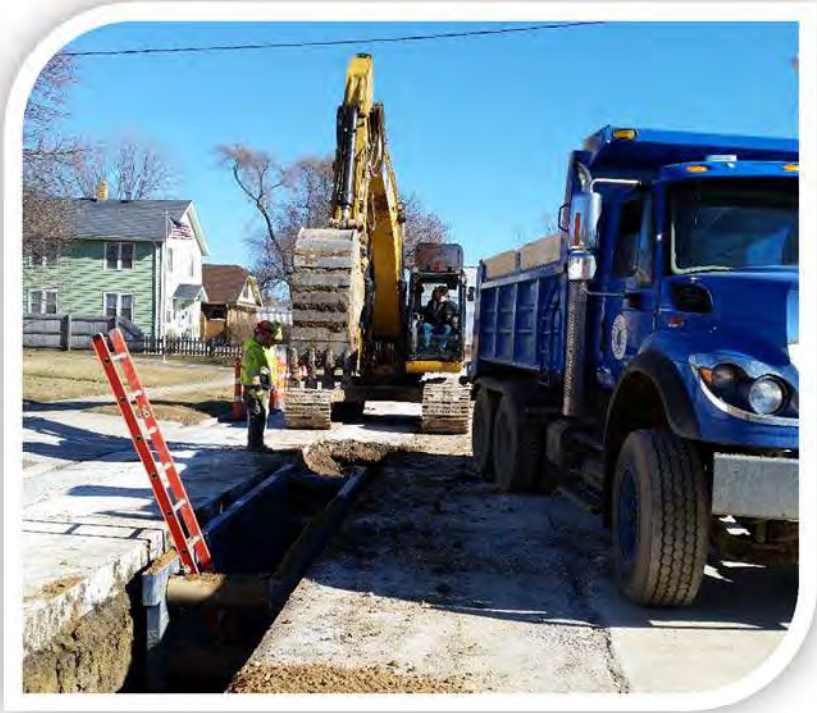
KWU distribution crews worked on ten water main relay projects during 2017 installing 6,589 feet of new water main
