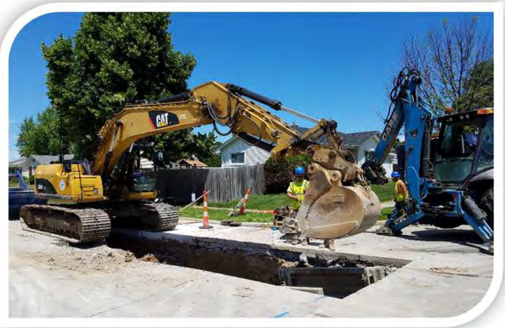
KWU distribution crews worked on ten water main relay projects during 2017 installing 6,589 feet of new water main
