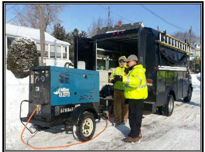
211 frozen water service laterals were thawed
