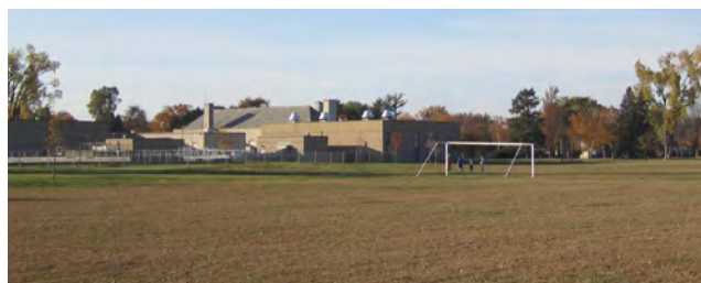
Wastewater Treatment Plant (SAA)
