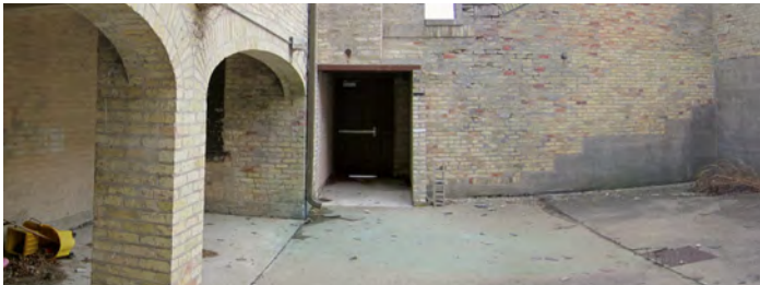
Bath House South Courtyard (Engberg Anderson)
