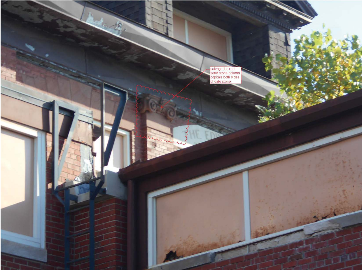
Item 8: Column Capital on both sides of the date stone.
