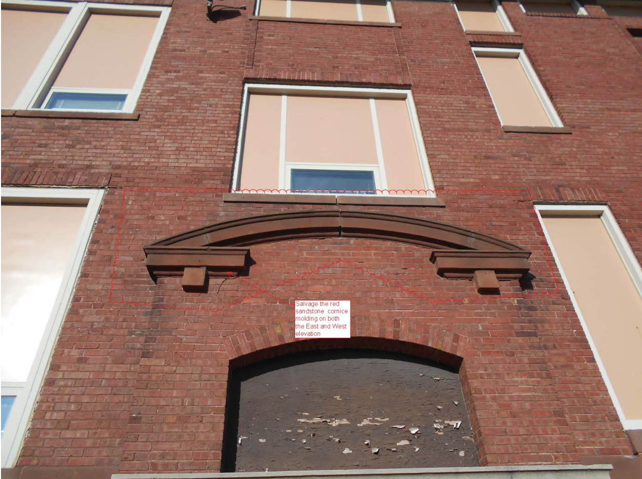
Item 3: The red sandstone cornice molding above the entries on both the East and West entries.
