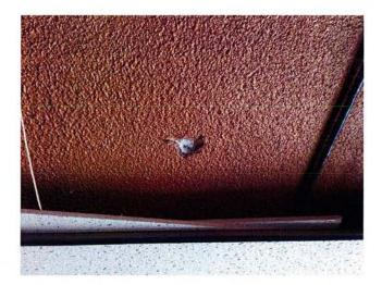
8. Sample 9109-011 location, spray-on sound proofing above suspended ceiling in bar area.
