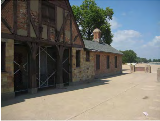
Image 4 – East side of the bathhouse – May 2010
