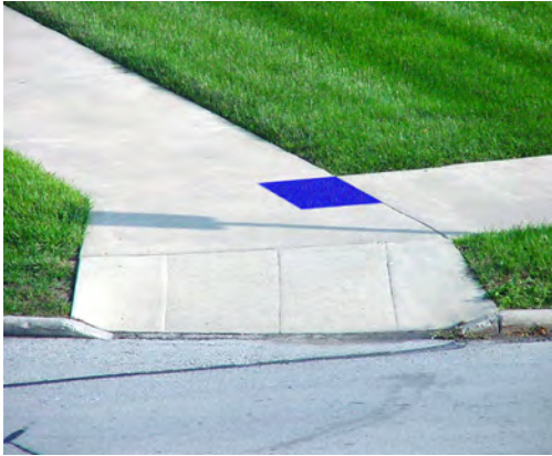
Figure 44. The simplest way to color-code sidewalks is to add a square of color near intersections.
