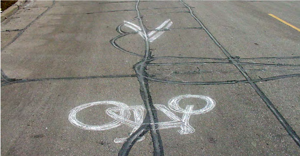
Figure 5. Shared-use lane markings can designate a bicycle route without a segregated bicycle lane. The pavement markings are placed to leave adequate space for vehicular traffic, parked cars and bicyclists.
